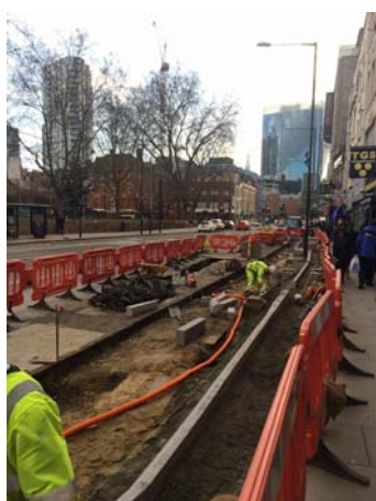
Cycle Superhighway Route 2 Upgrade - installation of the new segregated kerbs
