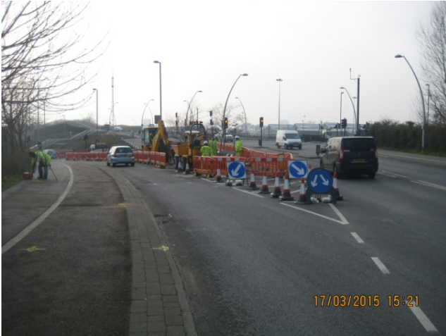
Ruckholt Road scheme in Waltham Forest, to complete mid 2015
