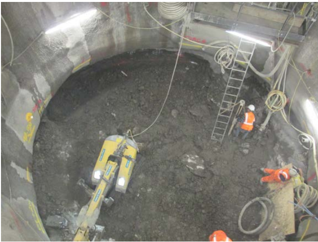
Vauxhall station shaft excavation
