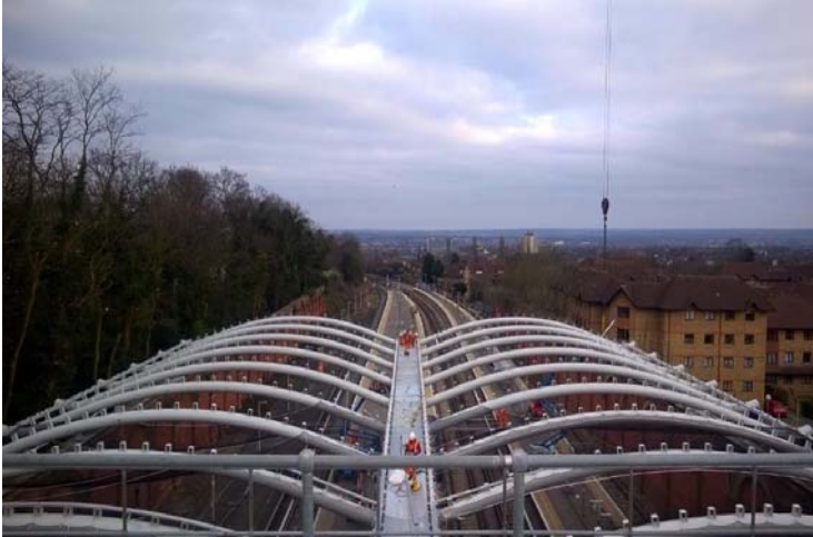
Installation of the gull-wing canopy over Crystal Palace Station
