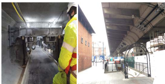
Internal deviator steelwork External post tension cable installation
