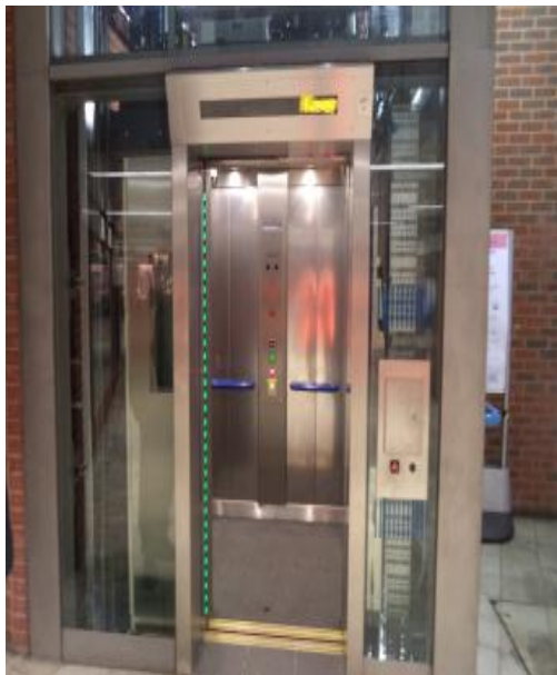
Completed lift at West Ham station
